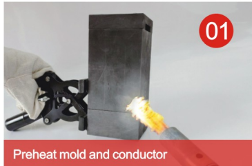
Preheat mold and conductor
