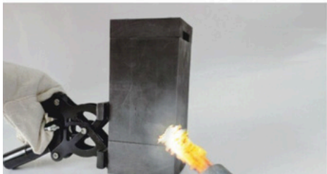
Preheat mold and conductor
